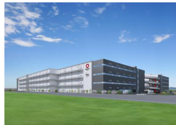
DPL Sakado (Saitama Pref.) Multi-tenant logistics facility is largest by Daiwa House
