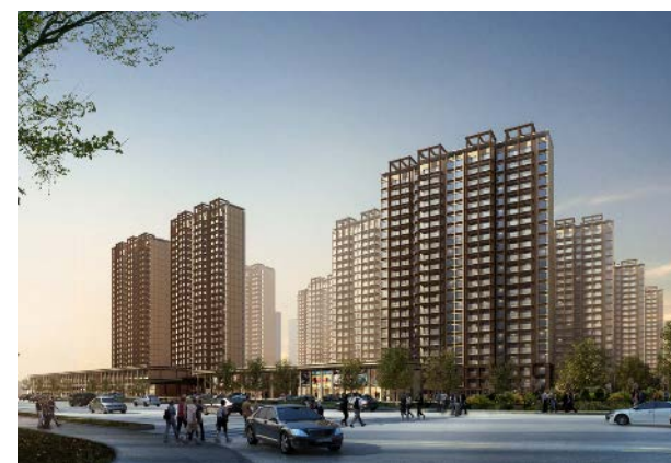
Nantong Project (Jiangsu Province) First large-scale condominium development in China in 6 years
