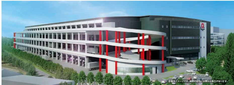
DPL Nagareyama (Chiba Pref.) Multi-tenant type logistics facility
