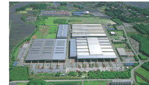
Tochigi Ninomiya Factory, which received the highest grade S certification from the Minister of Land, Infrastructure, Transport and Tourism in 2019
